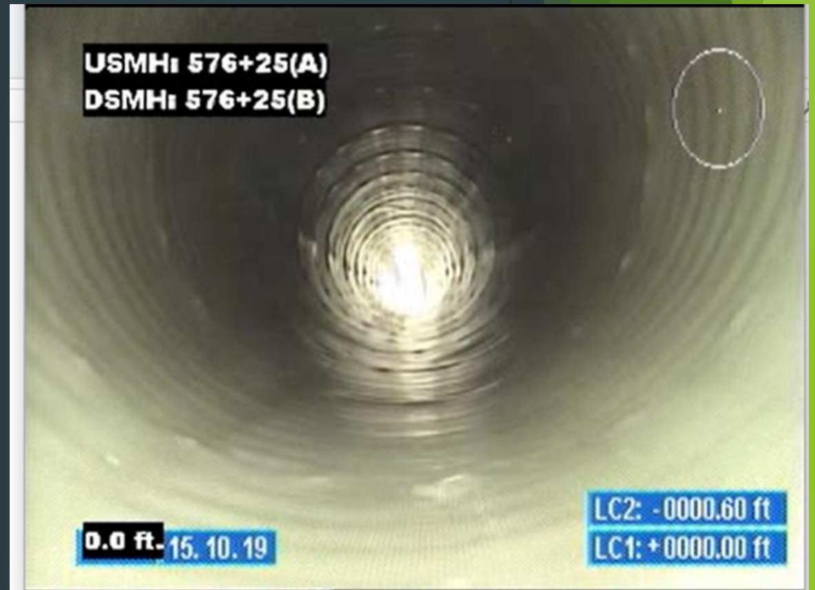
After Installation of Liner
