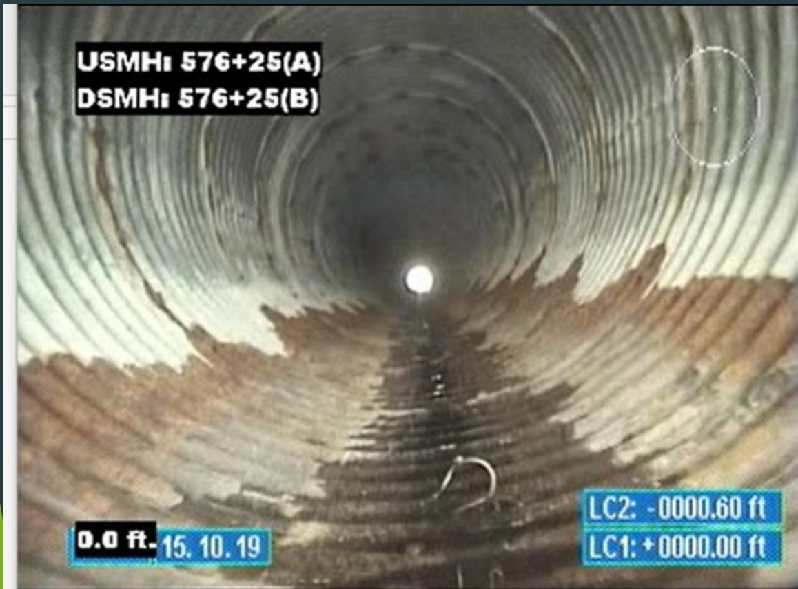
Before Installation of Liner
